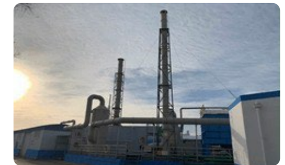
Collection and treatment of foul gas from the sewage station in the High-tech Park to ensure that no odorous gas escapes from the sewage station
