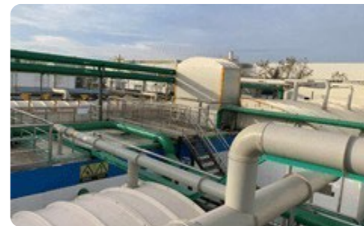
Collection and treatment of foul gas from the sewage station in the High-tech Park to ensure that no odorous gas escapes from the sewage station
